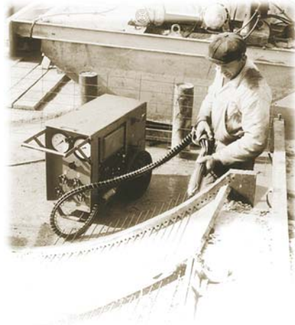
Production of HP roof shells at the end of the fifties
